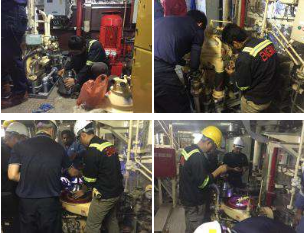
Testing, Commissioning & Harbour Acceptance Trial (HAT) F.O & L.O Purifier onboard RMN Training Vessels GAGAH SAMUDERA and TEGUH SAMUDERA.
