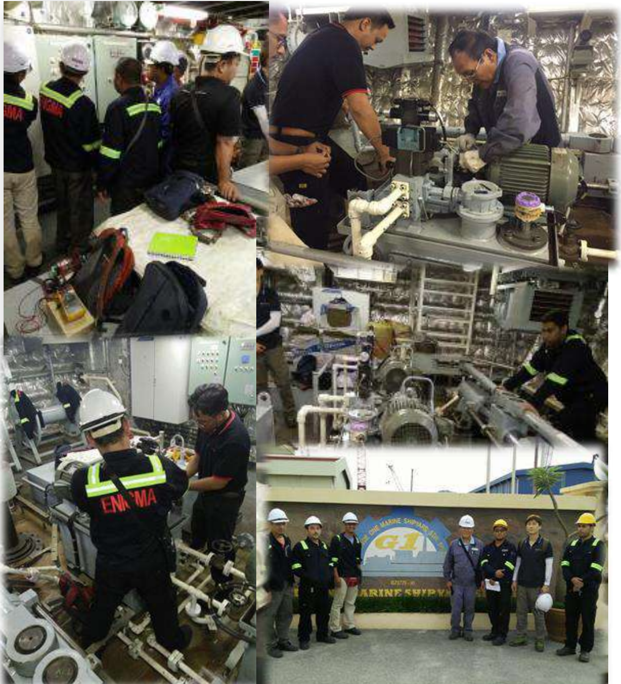
Testing, Commissioning & Harbour Acceptance Test (HAT) ARIM Steering Gears at Grade One Marine Shipyard (GOMS)
