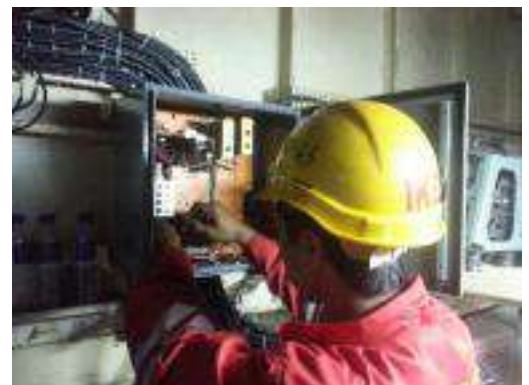
Echo Sounder Installation Work
