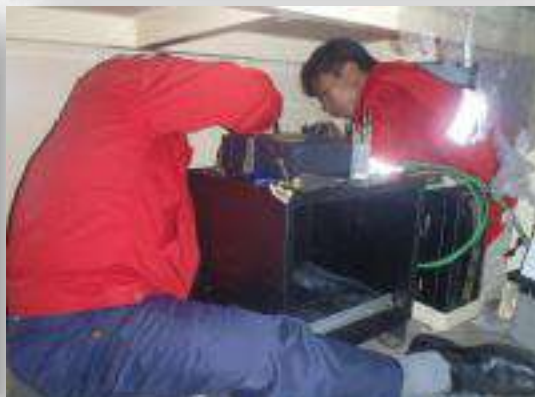
CABLING & TERMINATION WORKS
