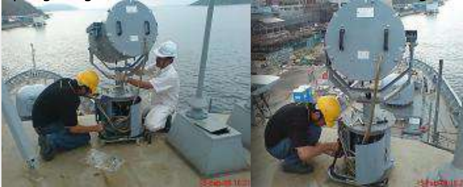
Vessel Search Light and Controller Servicing & Test
