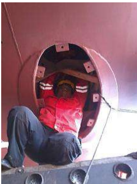
PREPARATION FOR THE INSTALLATION OF CATHODIC PROTECTION ZINC ANODES
