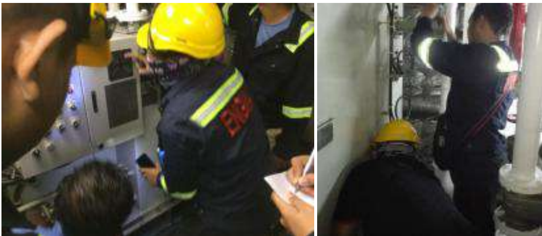
Testing, Commissioning & Sea Acceptance Trial (SAT) Sewage Treatment Plant onboard RMN Training Vessel GAGAH SAMUDERA.
