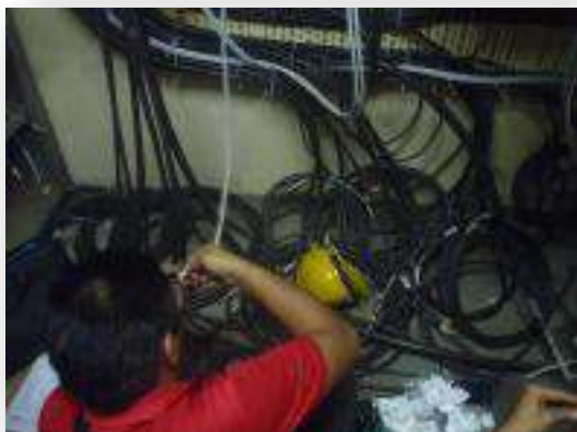
CABLES LAYING MARKING WORKS
