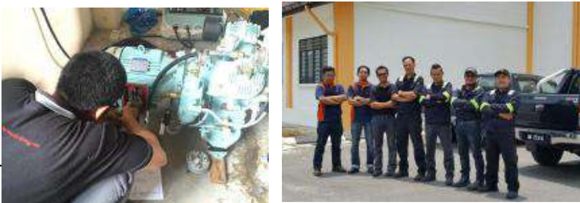
Testing, Commissioning & Supply Marine Air Compressor at Kolej Vokasional Pasar Gudang
