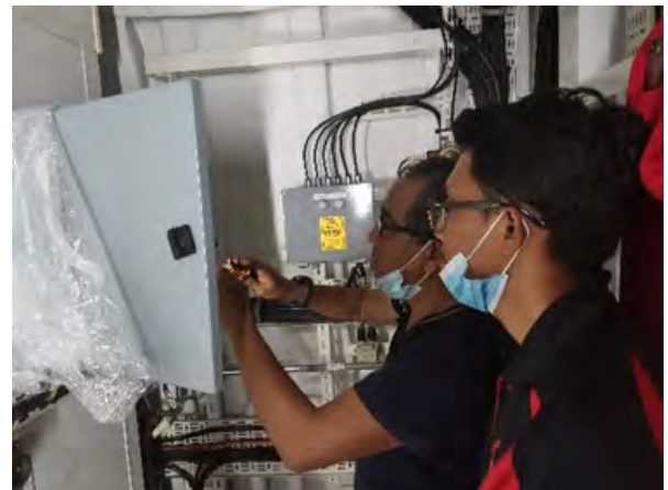
CABLING & TERMINATION WORKS
