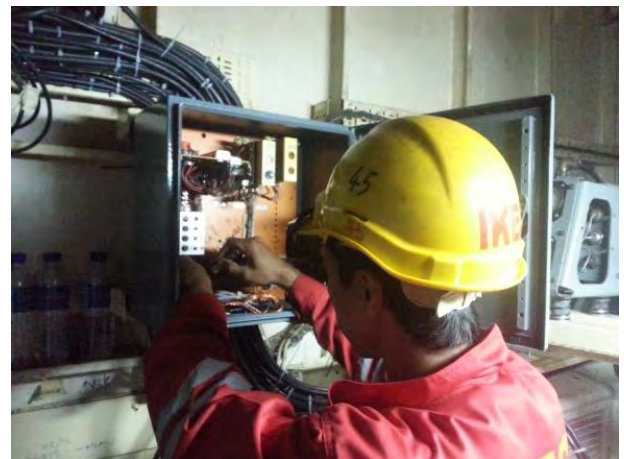
ECHO SOUNDER INSTALLATION WORK
