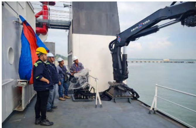
SETTING TO WORK AND COMMISSIONING FOR CRANE
