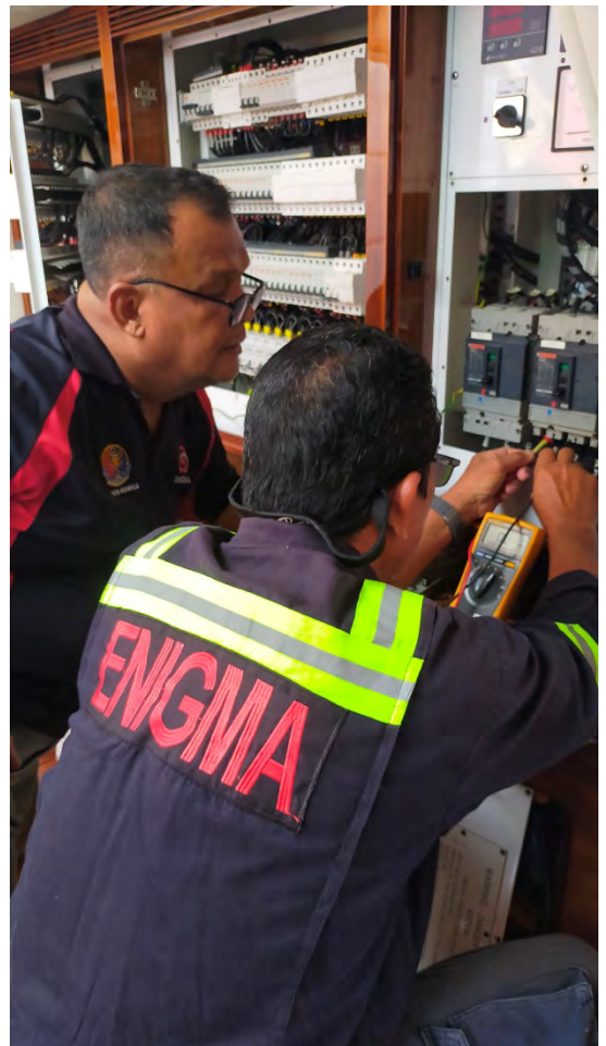
INSULATION AND CONTINUITY TEST
