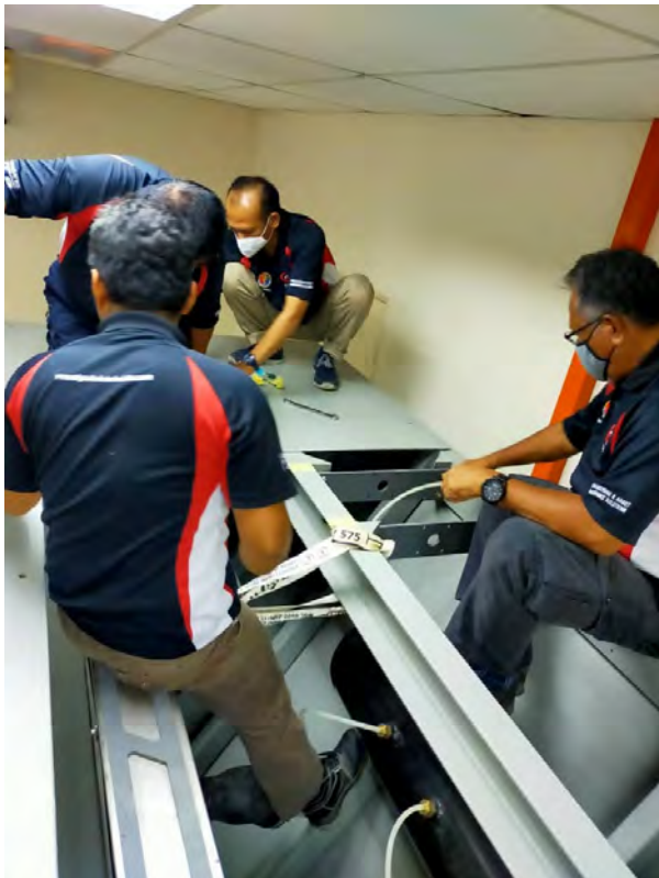
INSTALLATION OF ACTUATOR
