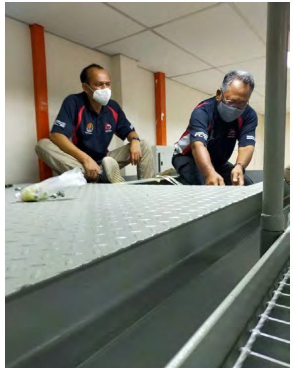
REMOVAL OF EQUIPMENTS
