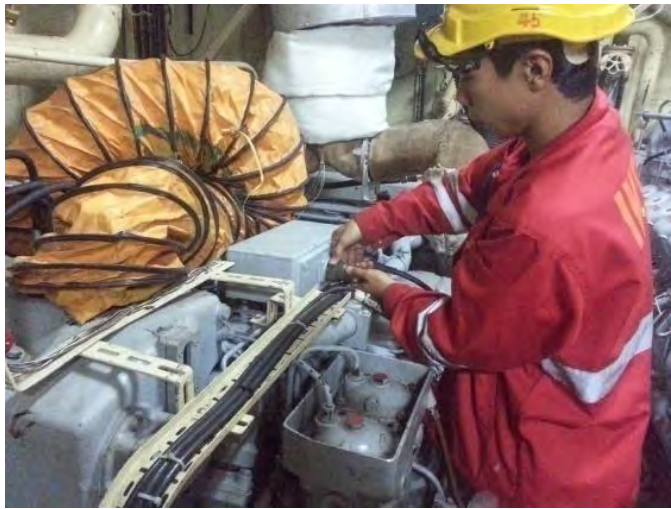
SHIP LIGHTING DISTRIBUTION BOX AND CONTROLLERS SERVICING & TEST
