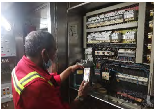
CABLES LAYING MARKING WORKS
