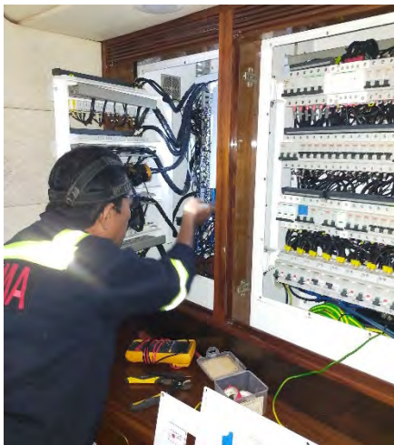
SWITCHBOARD VISUAL INSPECTION
